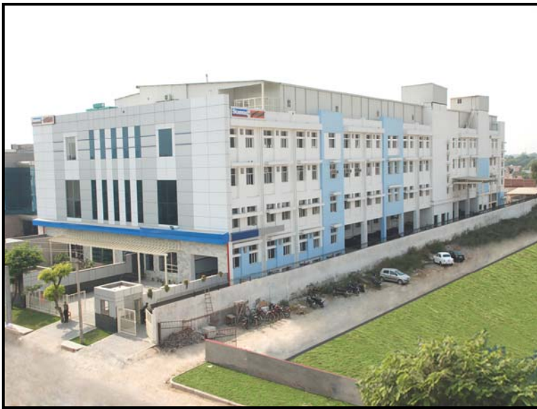
Plant III – Gurgaon : Stainless Steel Wires & Speciality Coatings, Fire & Anti - Corrosion
