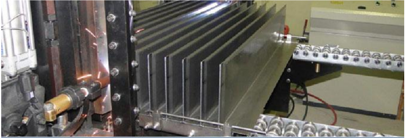
WELDING PROCESS OF CORRUGATED WALLS
