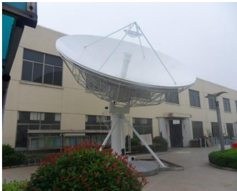
9.0m Earth Station Antenna
